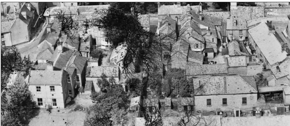
Fig. 12: Aerial photograph of 1932 showing The Cedars (left foreground) from the north-east. This image clearly illustrates the east and rear extension works of the Victorian period. [Detail of EPW039256 JUL-1932 © Historic England Archive (Aerofilms Collection)]
