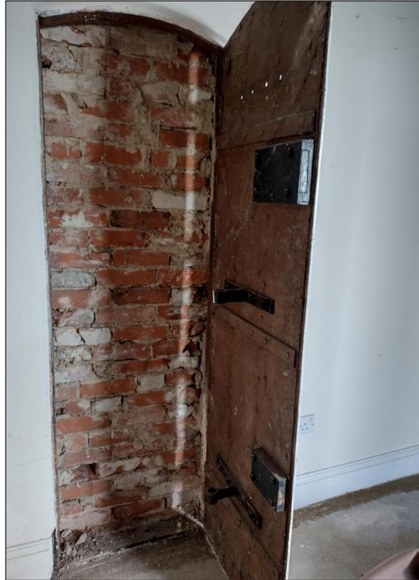
Fig. 63: The steel door which once joined the single-storey office building with the savings bank at 1 New Road. It was probably bricked up after the Second World War. [© North Norfolk District Council]
