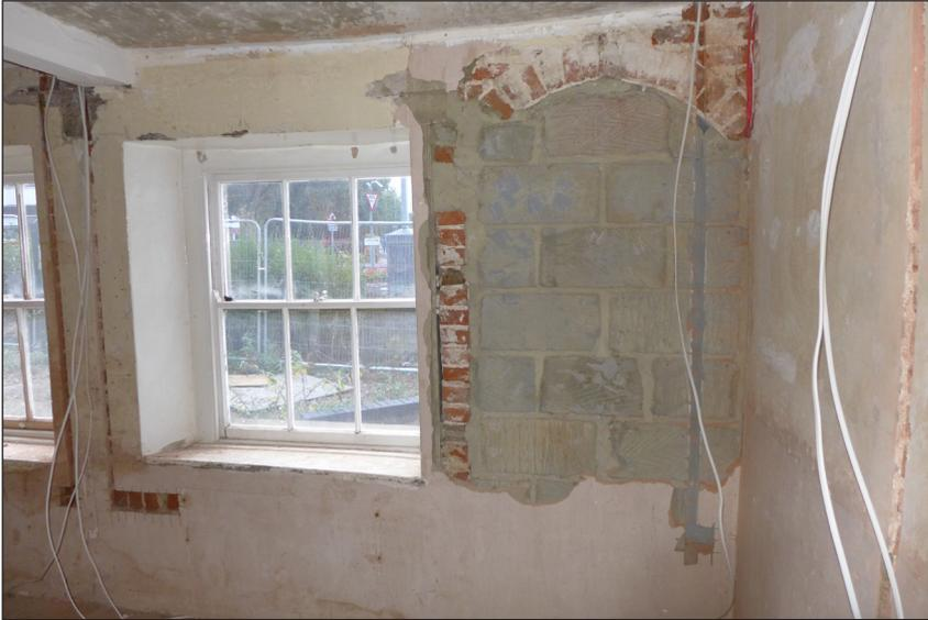
Fig. 59: The arched doorway opening at the south-west of the kitchen (G.11). This was probably original to the late 18th-century phase and was blocked in the 1990s. It formed a service entrance, accessed from the street via an enclosed part of the forecourt. [Emily Cole © Historic England]
