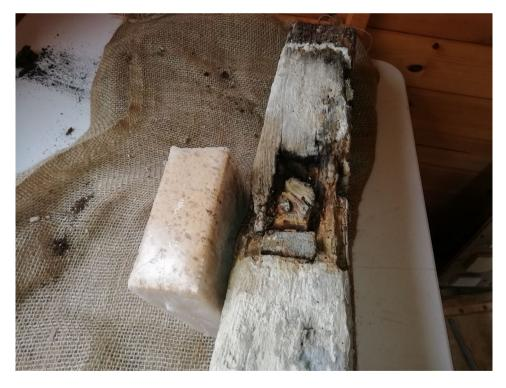
*Figure 3:* Ex situ *lintel showing mortice from a former role (photograph Martin Bridge)*
