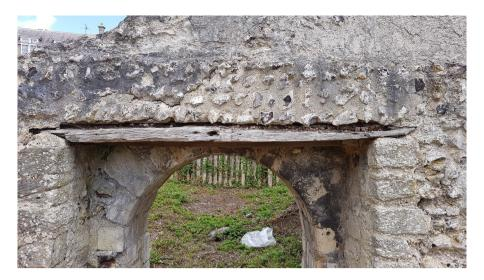
Figure 2: Photograph of the lintel in position over a doorway (photograph Maria Buczak)
