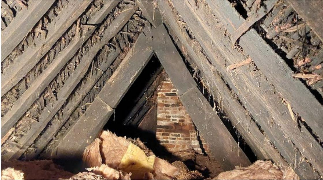
*Figure 2a: Cruck truss 2 showing north face (note how each blade is made up of an upper and lower piece) (photograph Robert Howard)*
