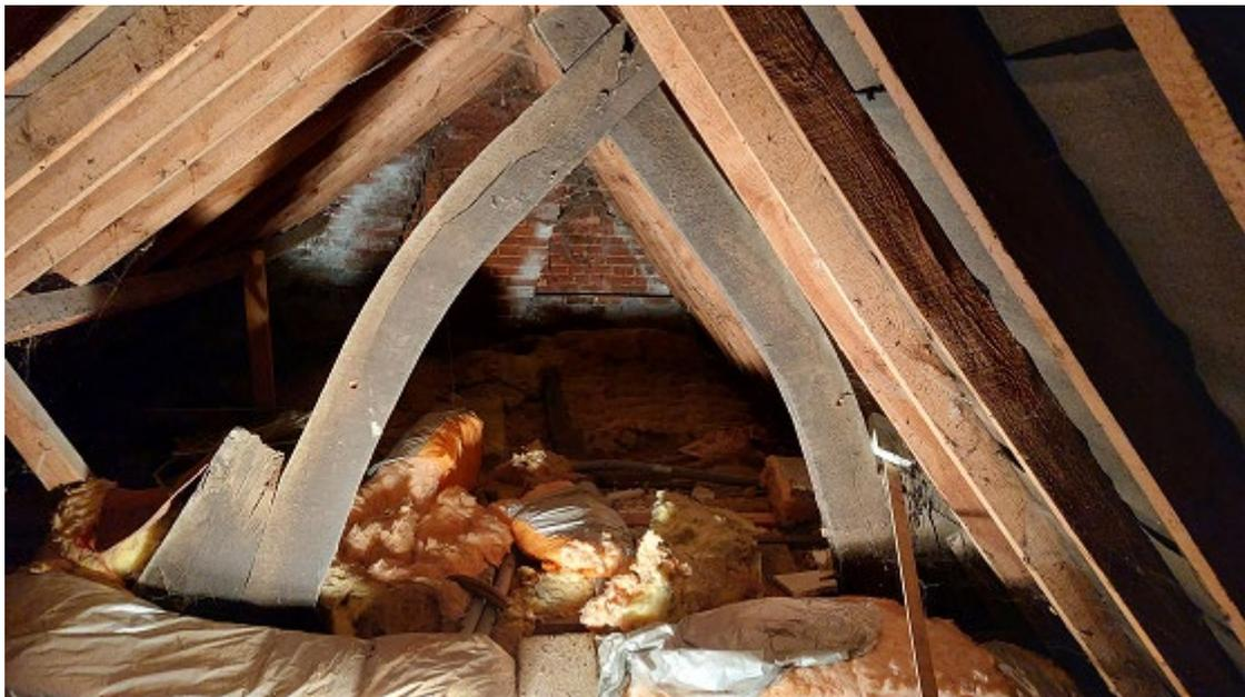
*Figure 2b: Upper section of cruck truss 4 showing north face (photograph Robert Howard)*
