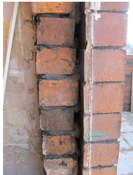
Figure 5: Removal of the door frame revealing a cavity in the wall
