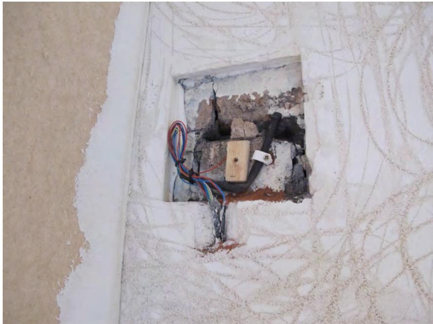
Figure 28: Relative humidity/temperature and resistance sensors fixed on the wall prior to the installation of internal wall insulation
