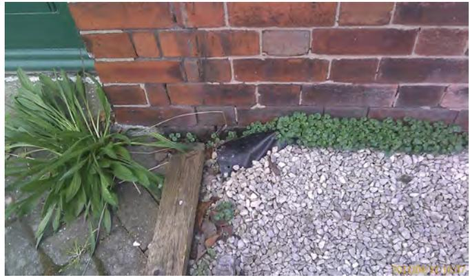
Figure 7: Vegetation at the base of the front elevation
