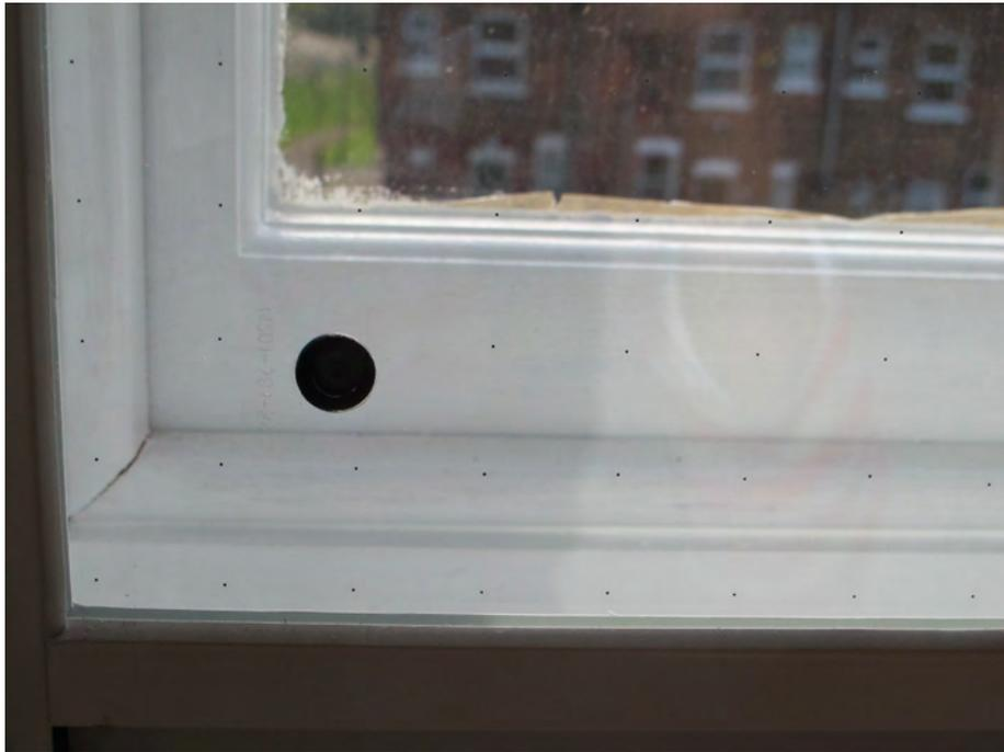
Figure 25: Detail of the slim profile vacuum glazing
