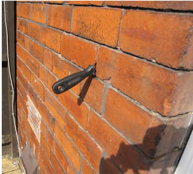
Figure 3: Deteriorated mortar joints
