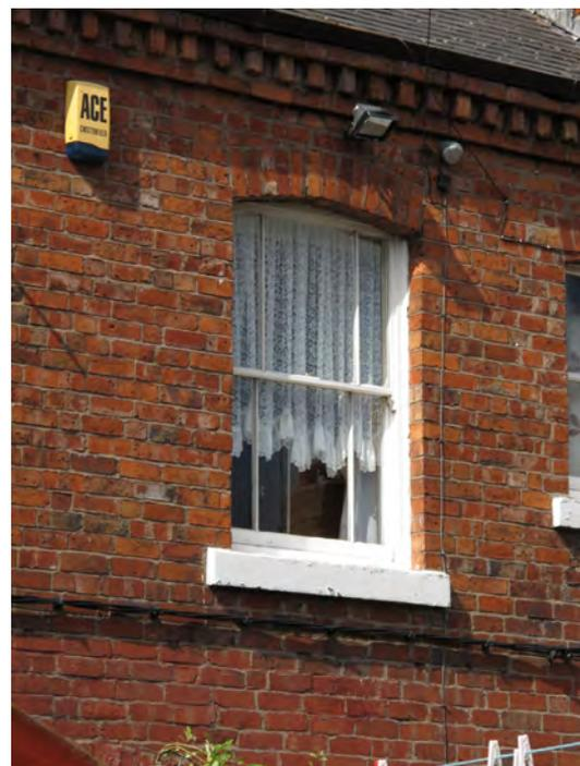
Figure 11: Original timber sash window
