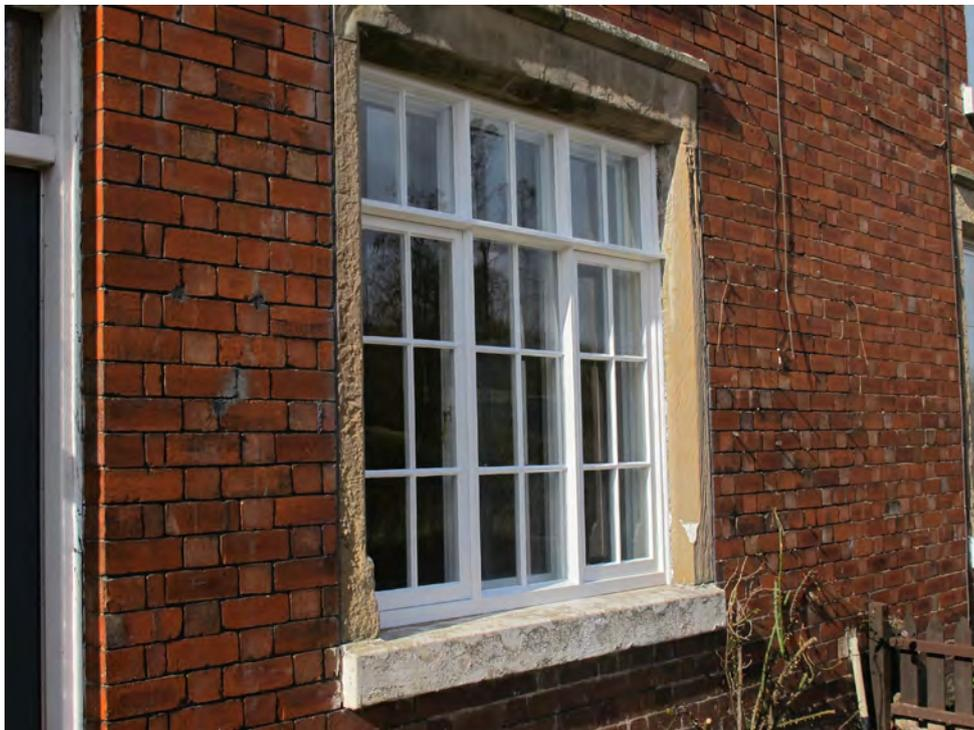
*Figure 22: Restored casement window on the front elevation*
