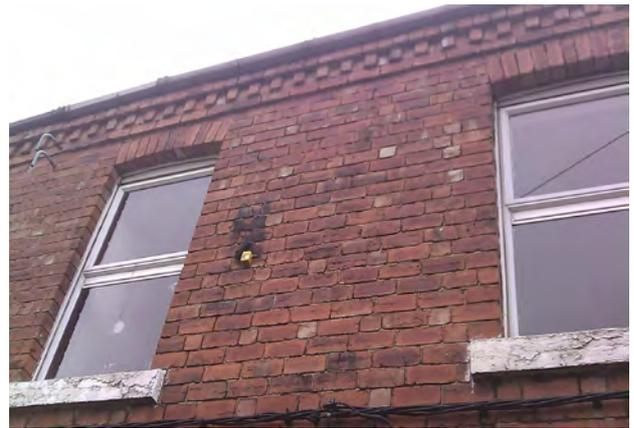
Figure 13: Plastic coated single glazed aluminium window on the rear elevation
