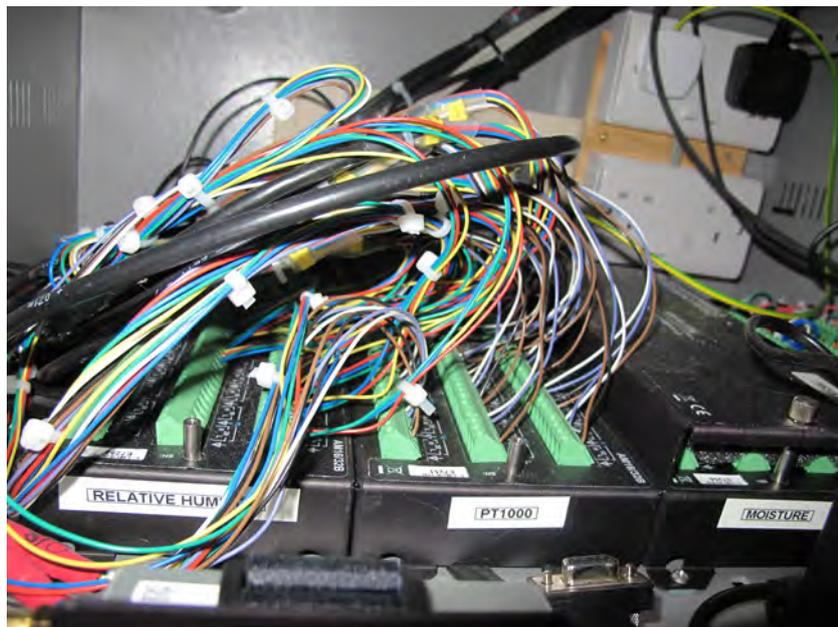
Figure 29: Data loggers hard wired to sensors installed in the house
