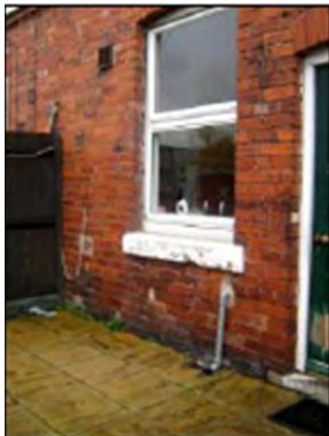
Figure 8: Irregularly laid paving slabs at the rear of the house channelling water to base of the rear elevation
