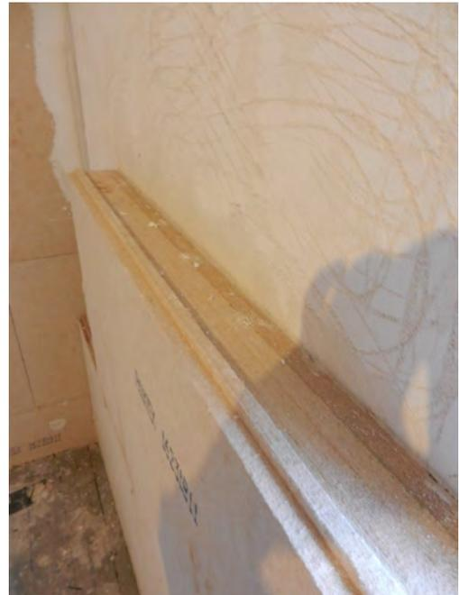
Figure 21: Lime plaster sandwich of the 100mm wood fibre insulation
