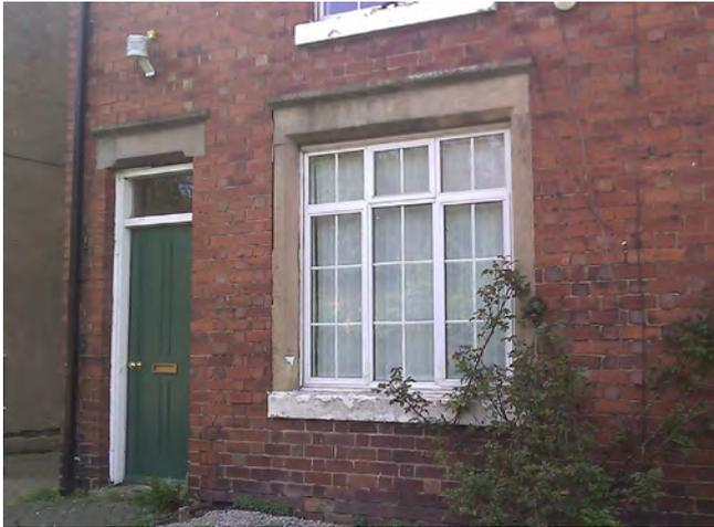
Figure 12: Plastic coated double glazed aluminium window on the front elevation
