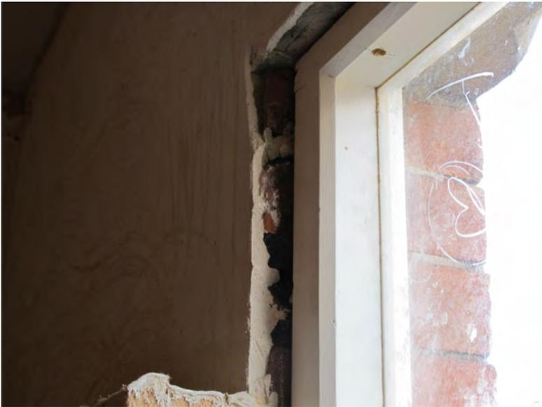
Figure 20: Varying thickness of the bonding coat of lime plaster
