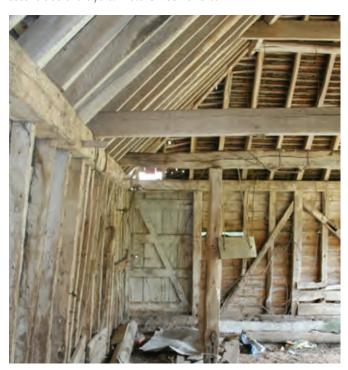
Shelter sheds usually provided shelter for cattle held loose in a yard but in the east of the region in particular open-fronted sheds could also be used to house tethered beasts. Any stall partitions have usually been removed but evidence of such use can survive including the presence of doors in the gable ends which gave access to a feeding passage along the back of the shed. Photo © Bob Edwards
