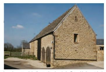
In regular courtyard plan farmsteads, as here in the Cotswolds, the cart shed often forms part of one of the ranges. Its function is identified by it having its openings on the external elevation of the range, facing onto the road which passes through the farmstead. Photo © Bob Edwards
