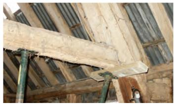
Evidence for vertical boarding. The butt-edged boards were set into a rebate on the frame so that the cruck blade and the tie beam were exposed. Photo © Bob Edwards
