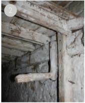
I Lofted stables often have a hay drop along one side allowing hay from the loft to be lowered into hay racks on the ground floor. Here wattle hurdles have been used to block the hay drop.
