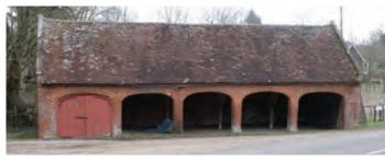
A brick-built cart shed in the South Hampshire Lowlands with one bay having doors so that small implements could be stored securely. Whilst most cart sheds were open-fronted, some examples retain evidence for having had doors to one or more bays in the form of pintel hinges in the posts. Photo © Bob Edwards
