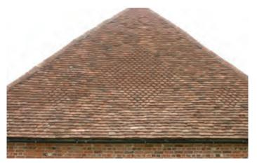
Plain clay tiles were being used to replace thatch in clay areas from the late 17th and early 18th century. Here the tiles include a pattern to the hipped end of a barn facing the roadside. Photo © Bob Edwards
