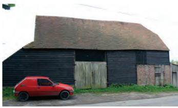
Stables could form part of combination barns from the medieval period. Here the stable element in the end bay has been rebuilt in brick. Photo © Bob Edwards
