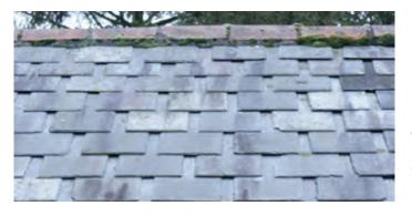
Welsh slate became readily available with the growth of the railways. Their lighter weight allowed for a reduction in the size of timbers need for roof construction. On estate buildings it is not uncommon to find slates being laid 'economically' to reduce the number of slates needed as so reduce the costs. Photo © Bob Edwards
