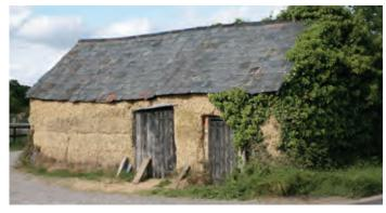
A small earth-walled building in the New Forest. The 'lifts', the phases of building up of the clay walls can be seen as horizontal bands of clay with slightly different textures and amount of small stones in the clay. Photo © Bob Edwards
