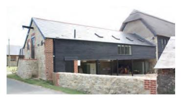
Cart shed in the Isle of Wight with a first-floor granary, accessed by steps at the gable end. This range retains the arm of the hoist used to raise and lower the sacks of grain. Photo © Bob Edwards
