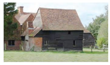
A rare survival of a detached kitchen to the rear of a High Weald farmhouse. Such buildings will often have smoke-blackened roof timbers to at least part of the roof and may have been partly floored. The stack at the gable end is a later addition. Photo © Steve Podd, FWAG
