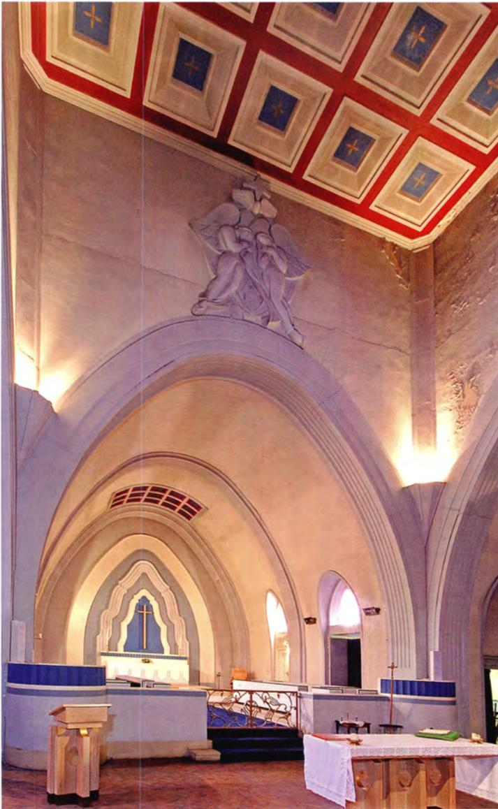
Figure 38 At St Christopher's, Norris Green, Bernard Miller used a plaster-coated steel frame to create the parabolic arches of its striking interior, quite unexpected from the severe angularity of its exterior. [DP034198]
