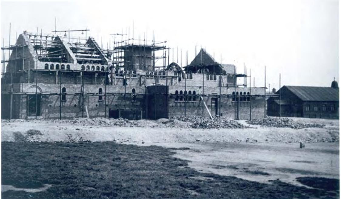
*F L Charlton also designed St Cross, Middleton, and this view taken in 1935 shows how it was constructed using a series of concrete arches. To the right may be seen the temporary building that preceded it, typical of how many suburban churches started life. (Courtesy of St Cross)*
