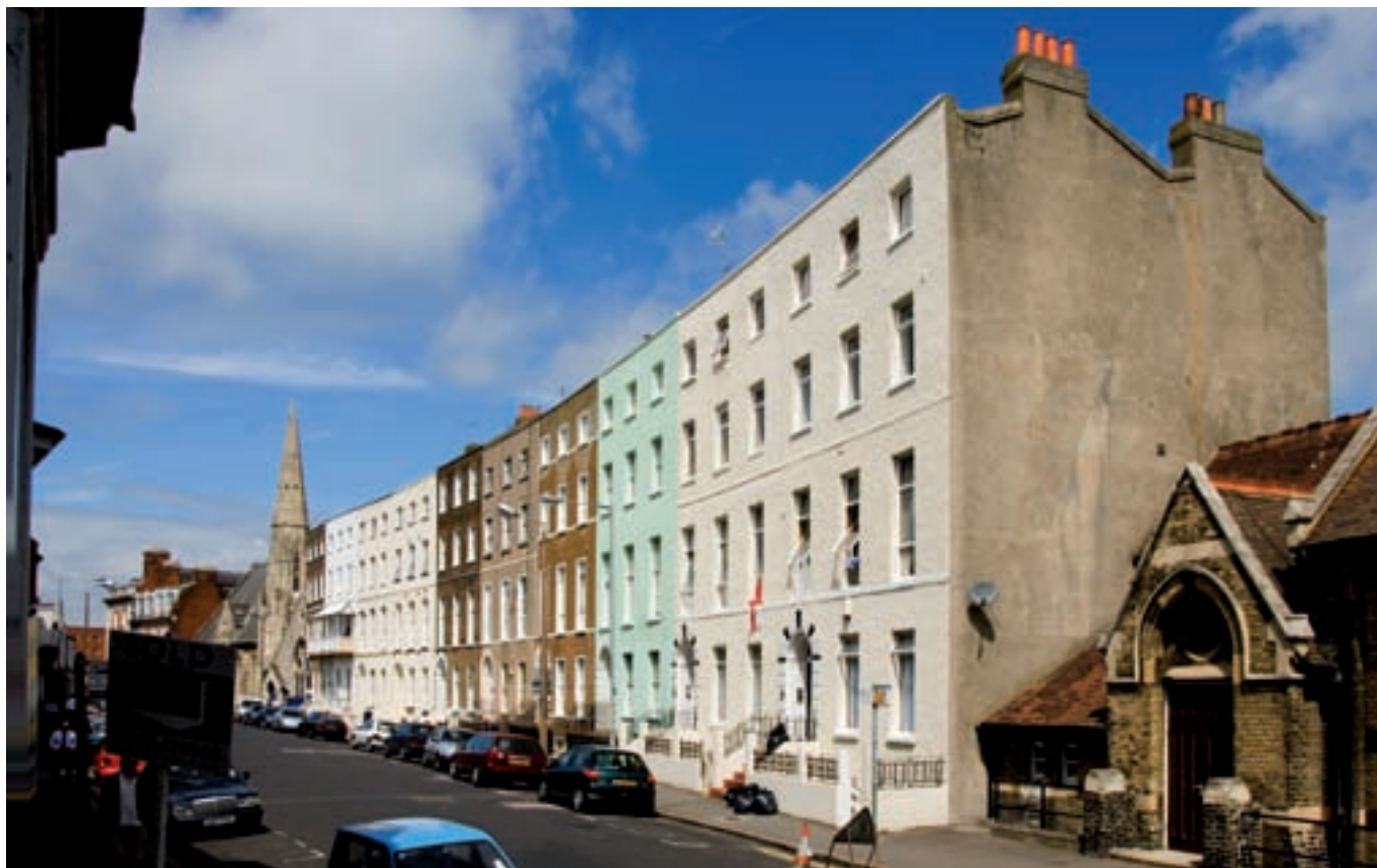
Figure 32 The double-pile, four-storied houses of Union Crescent are typically Georgian in form: each house is three bays wide, with sash windows diminishing in height storey by storey. They remained popular high-class residences into the mid-19th century. [DP026090]
