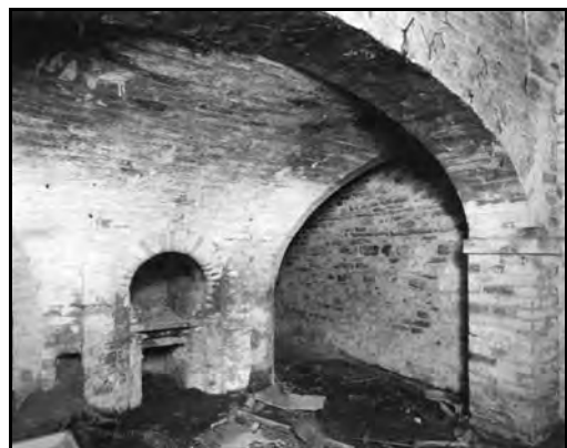
46. Malt kiln furnace - Burghley Park, Cambridgeshire. [BB95/02438]
