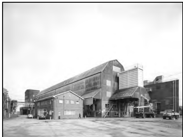
79. Saladin Box Maltings, Gainsborough, Lincolnshire. [AA98/03358]
