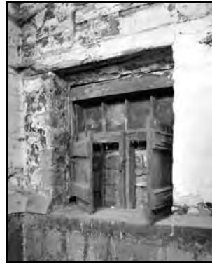
33. Anchor Brewery, Boroughbridge, North Yorkshire. [AA98/02214]
