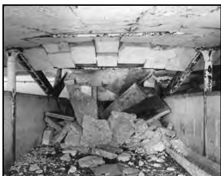
63. Midford, Clearbrook, North Somerset. [BB96/10269]
