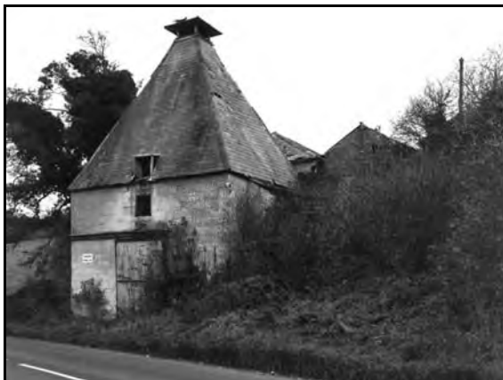
50. Exterior of Malt Kiln, Clearbrook, Midford, Somerset. [BB96/10262]
