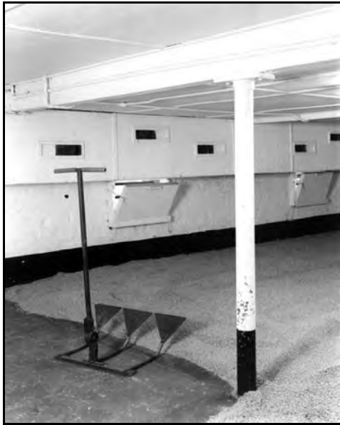
37. Air conditioning unit - East Dereham, Norfolk. [BB93/10023]
