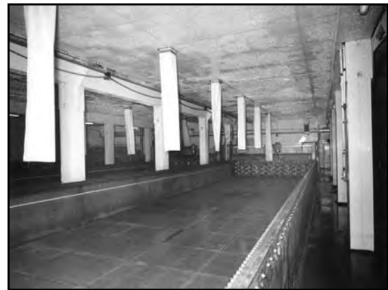
30. Saladin boxes - Gainsborough, Lincolnshire. [AA98/03369]
