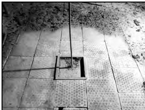
43. Perforated Kiln Tiles, Warminster Maltings, Wiltshire. [BB95/05264]
