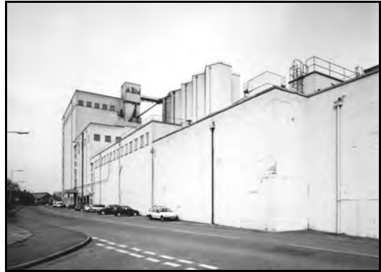
71. Pneumatic maltings, Louth, Lincolnshire. [AA98/03378]
