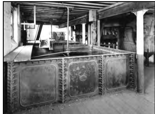
20. Top cast iron steep - hopper bottomed – Malthouse No 4. Weymouth. [BB95/08086]
