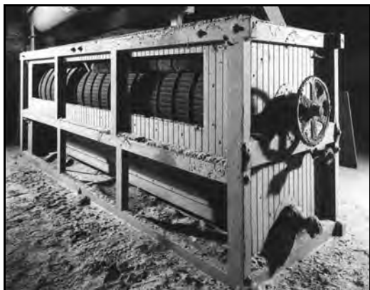
51. Grain Cleaner, Downing's Malthouse, Gloucester. [BB94/17203]
