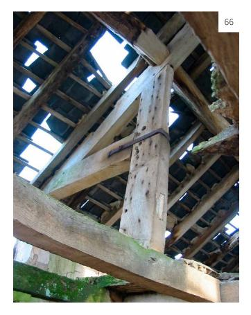
Image 66 Without a weatherproof covering this roof structure will rapidly decay.
