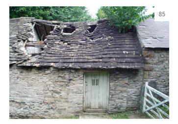
Image 85 These stone slates had been covered in bitumen preventing their re-use.
