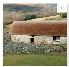
**Image 33: Thatch** was historically the most widespread material for roofing farm buildings, although its method of application varied from region to region and according to the available raw material. Long straw and combed wheat reed (also called Devon reed) were the most common, but heather and water reed were also used in areas where they grew naturally.
