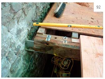
Images 91 and 92 Joist end repairs using steel T-sections.
