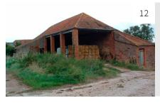
**Image 12: Hay-barns** were constructed in areas where large numbers of cattle were housed over winter. Metal-framed 'Dutch' barns (originally termed 'French' barns) date from the 1880s.
