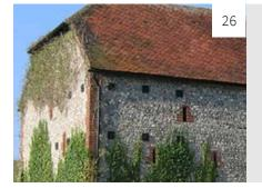
**Image 26: Flint** was used as a building material in chalk areas of eastern and southern England that lacked a better local form of building stone. Brick lacing courses provided extra strength and stability and brick dressings were used to form quoins and openings.
