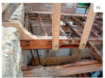
Images 93 and 94 New joist end scarfed onto an existing joist.
