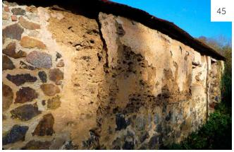
Image 45 Bird and bee damage to decayed cob walling.
