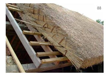
Image 88 Combed wheat-reed thatching in progress with the fixings visible.
