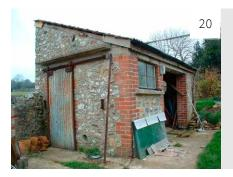
**Image 20: Dairies** may be attached to and part of the dwelling house. Rare examples will still have stone or slate shelves and stone or brick floors with good drainage. Less commonly, a channel will allow a through-flow of cooling water. Examples within model farms may also feature decorative tiling and even elements of gothic or *ferme ornée* design.
