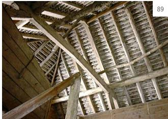
Image 89 Most roofs of farm buildings have no underfelt allowing the roof timbers to be well ventilated.
