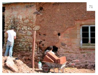
Image 71 Repairs underway to a stone and cob wall using lime mortar and new blocks of cob.
