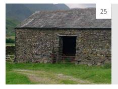
**Image 25: Stone** dominates the stock of farm buildings in many parts of the country, its use sometimes reflecting the status of the farm and its owner. Because each kind of stone has its own special properties, masons learnt to shape and bond the material in locally distinctive styles.
