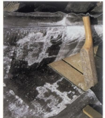
Figure 18 In this VWR, the AVCL terminates some distance short of the abutment. The lead nearby has corroded underneath, which is to be expected in the circumstances. Some condensate has also entered the lap and caused local corrosion.
