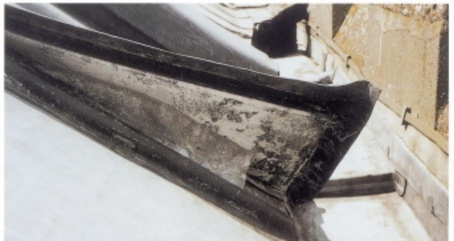
*Figure 16 This early example of a VWR was ventilated from side to side, rather than from bottom to top. ULC has occurred in the less well-ventilated area near the eaves between the two bottom vents.*
