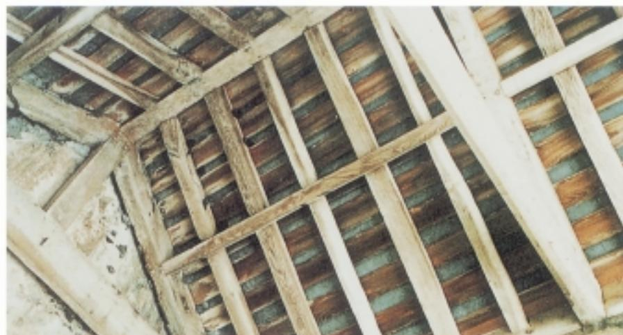
*Figure 20 A gap-boarded roof. Softwood gap boarding is common in the steeply-pitched roofspaces of medieval cathedrals. It is normally unsuitable mechanically for flat or shallow-pitched roofs. For a variety of reasons, these roofs tend to be relatively resistant to ULC and the construction can often be maintained without any modification. A pretreatment on the underside can help to avoid initial corrosion. See Section 6.*
