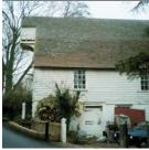
SITE NAME: Spring Valley Mill, Spring Valley C18 watermill, white weatherboarded over painted brick base. Beam engine circa 1873 now gone. Mill disused since Lane, Ardleigh 1930s. Machinery complete. Road elevation and lucam DESIGNATION: Listed Building grade II\* remain scaffolded. CONDITION: Poor OCCUPANCY: Vacant/not in use PRIORITY CATEGORY: C (C) OWNER TYPE: Private LIST ENTRY NUMBER: 1112053 Contact: Sheila Stones 01223 582716
