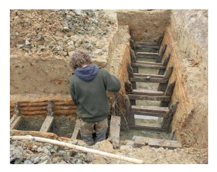
Excavations at 'Forward Cottage' in the Ypres Salient in 2005, provide a fascinating insight into the development of trench warfare inverted A frames in a British trench, designed to provide a dry and stable platform for wooden duckboards. This shows a level of detail beyond that which could be gleaned from documents © Peter Doyle
