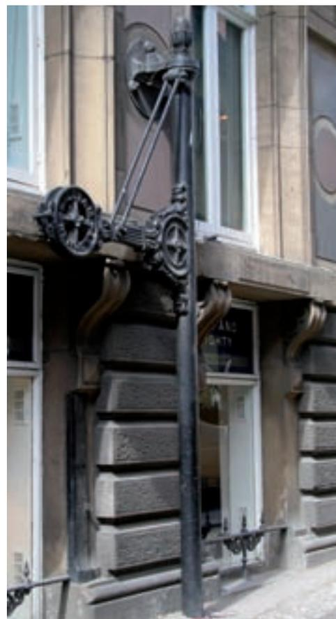
Figure 43 (above) *An unusually decorative cast-iron hoist in Hackins Hey, originally serving the basement of 11 Dale Street. [Joseph Sharples]*
