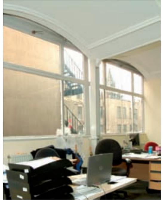
Figure 61 (above) *Glazed curtain walling to the courtyard elevation of Oriel Chambers, independent of the building's cast-iron frame. [DP28852]*
