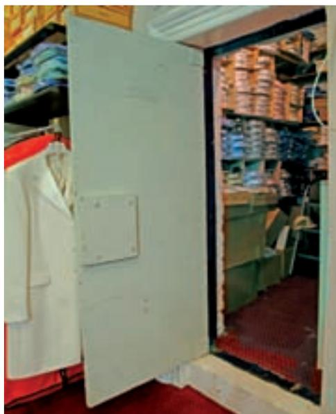
Figure 51 (above) Cast-iron door of a former safe or book case in Harrington Chambers, North John Street, now used as a stockroom by the current occupier, a men's outfitter. [DP28707]
