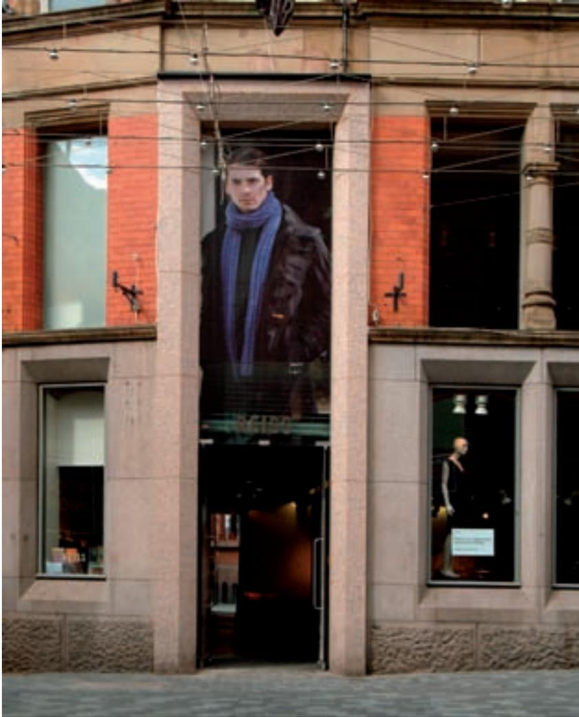
Figure 91 *Reiss, a fashion store in a converted 19th-century office building in Mathew Street. The new entrance matches the scale of the original building, and its narrow proportions echo the warehouse loading bays of neighbouring blocks. [DP28722]*
