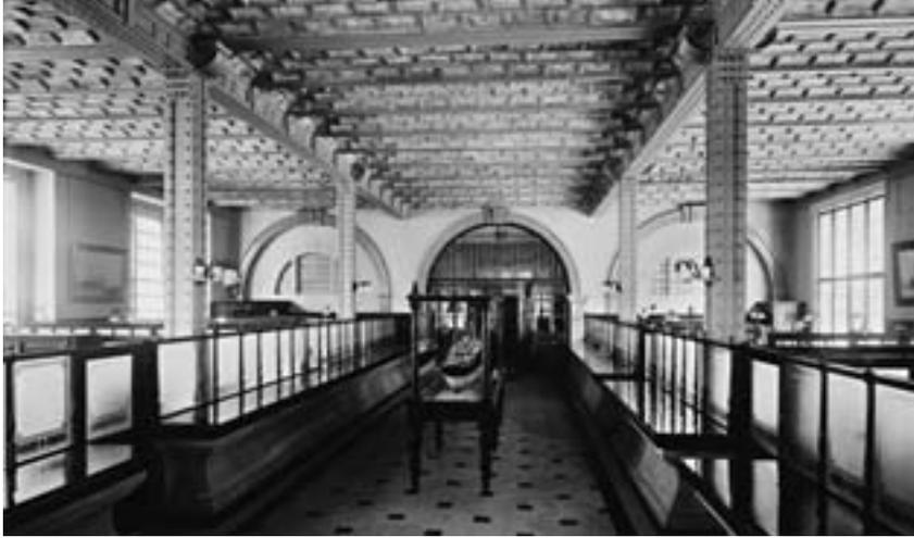
Figure 71 Former public office of the White Star Line building, James Street, 1895–8, by Richard Norman Shaw; photographed in 1898 by Bedford Lemere. The ceiling is fireproof, of terracotta panels held in a cast-iron frame. [NMR BL 14773]
