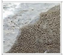
Visible water beading on impermeable surfaces such as glass or metal under certain conditions; wall feels cold and damp to touch; may be damaged finishes or signs of moisture problems (such as decay for timber affected by runoff)
