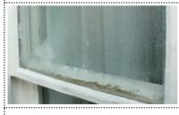
Significant condensation on the inside of the glass, occurring regularly; runoff staining below the window; decay of timber cill and horizontal members of windows, or corrosion of horizontal members and joints of metal windows
