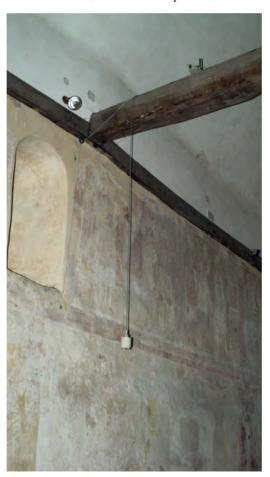
Most monitoring begins with equipment to measure temperature and relative humidity, often together with surface temperatures. Monitoring exterior and interior microclimates is also standard, as this more than any other comparison reveals how the building envelope is working. The weather station is a particularly useful tool, combining in a single unit the measurement of exterior temperature and relative humidity, rainfall intensity, sunlight, and wind.
