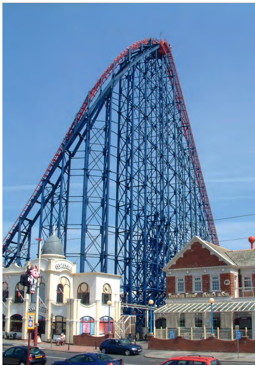
Figure 75 The Big One, a thrilling, mile-long ride, has a 235ft-high lift hill that propels the cars around at over 70mph. [DP022320]
