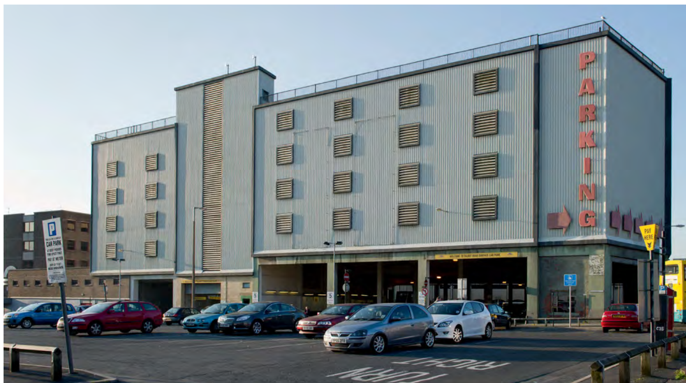
Figure 83 The original conception of the Talbot Road Bus Station and Car Park now seems commonplace, belying the innovation shown in the original structure of 1937–9. The exterior was re-clad in 1963. [DP119488]
