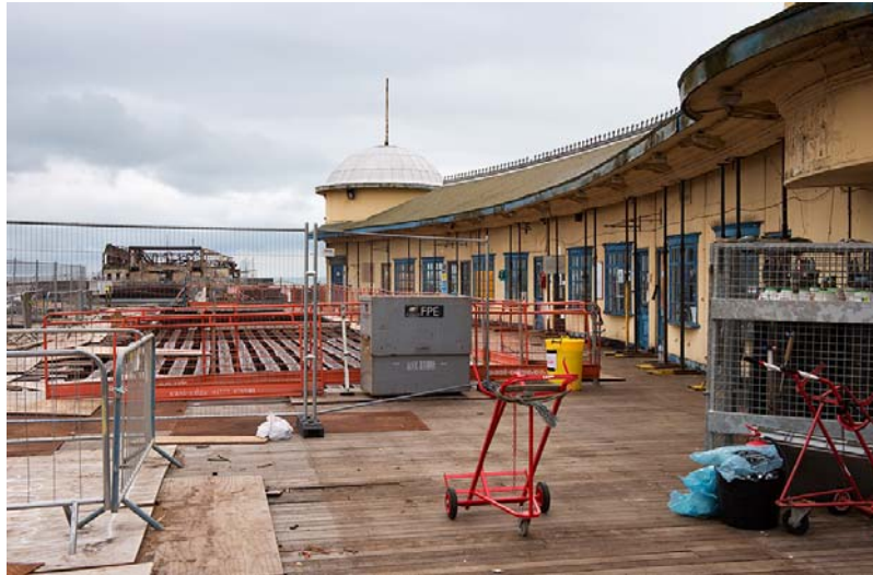
Work begins on the Pier © James Davies, English Heritage
